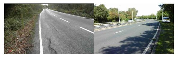
Asphalt Delamination on Concrete – This requires specialist repair works.
